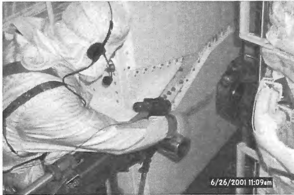
Figure 4. J-Hook operator measuring distance from trunnion to a closed passive latch with a tethered scale. Note the fall protection on the J-Hook operator.
